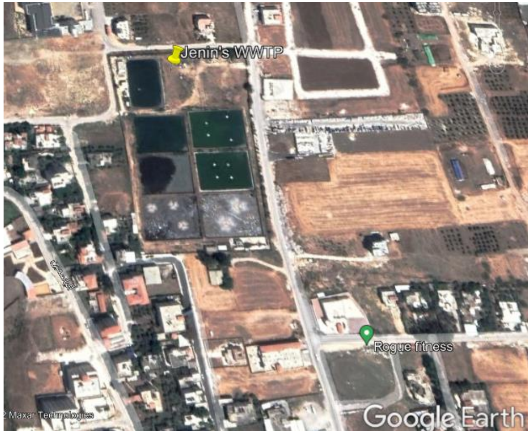
Figure 6. An aerial photo of Jenin’s WWTP (Google Earth Pro, 2022)
